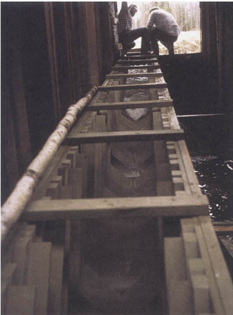
Figure 14. The Denil II fishway is a long chute with interior baffles to slow the water for fish passage. Photo by J.B. Kemper.
