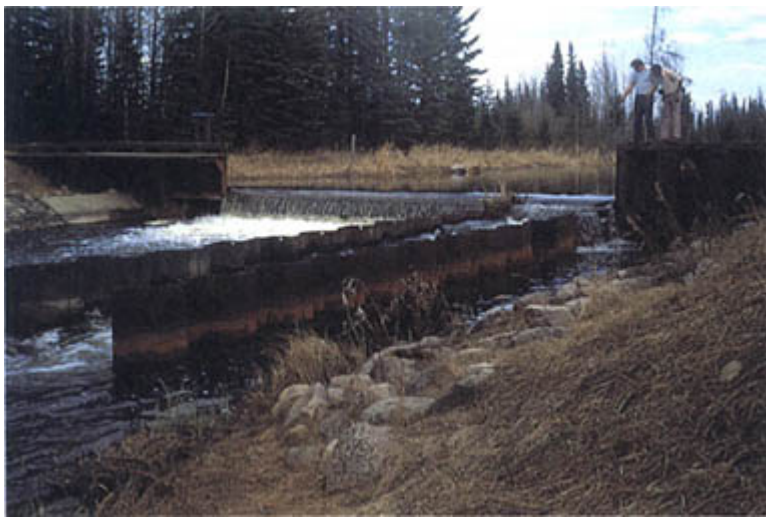
Figure 13. The weir on Steele Lake is a sheet-pile structure equipped with a step-pool fishway. Photo by J.B. Kemper.
